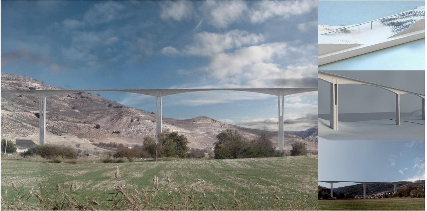
The structure is composed of 14 spans measuring 40.0m + 3 x 70.0m + 150.0m + 5 x 250.0m + 150.0m + 2 x 70.0m + 40.0m, reaching a total length of 1980.0m. The bridge is 24.0m wide so allowing the occupation of a dual carriageway.
